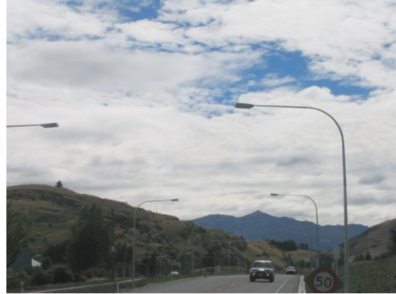
Streetlights near turnoff to Frankton Airport Note the horizontal arms supporting the fittings.
